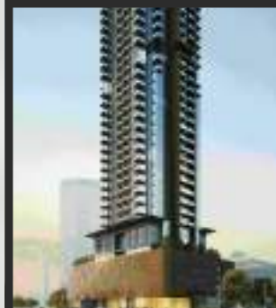
Seslia Tower JVT, Dubai
